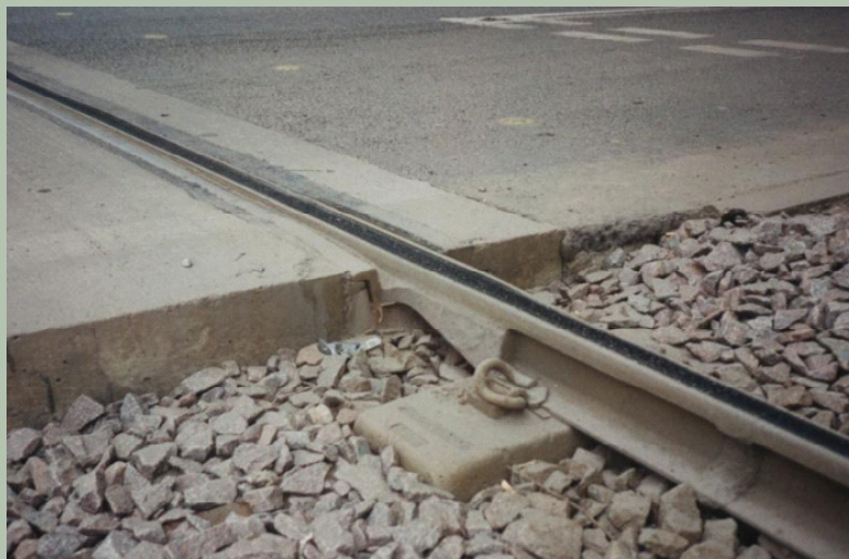
LR55 track in situ at Rotherham bus station
